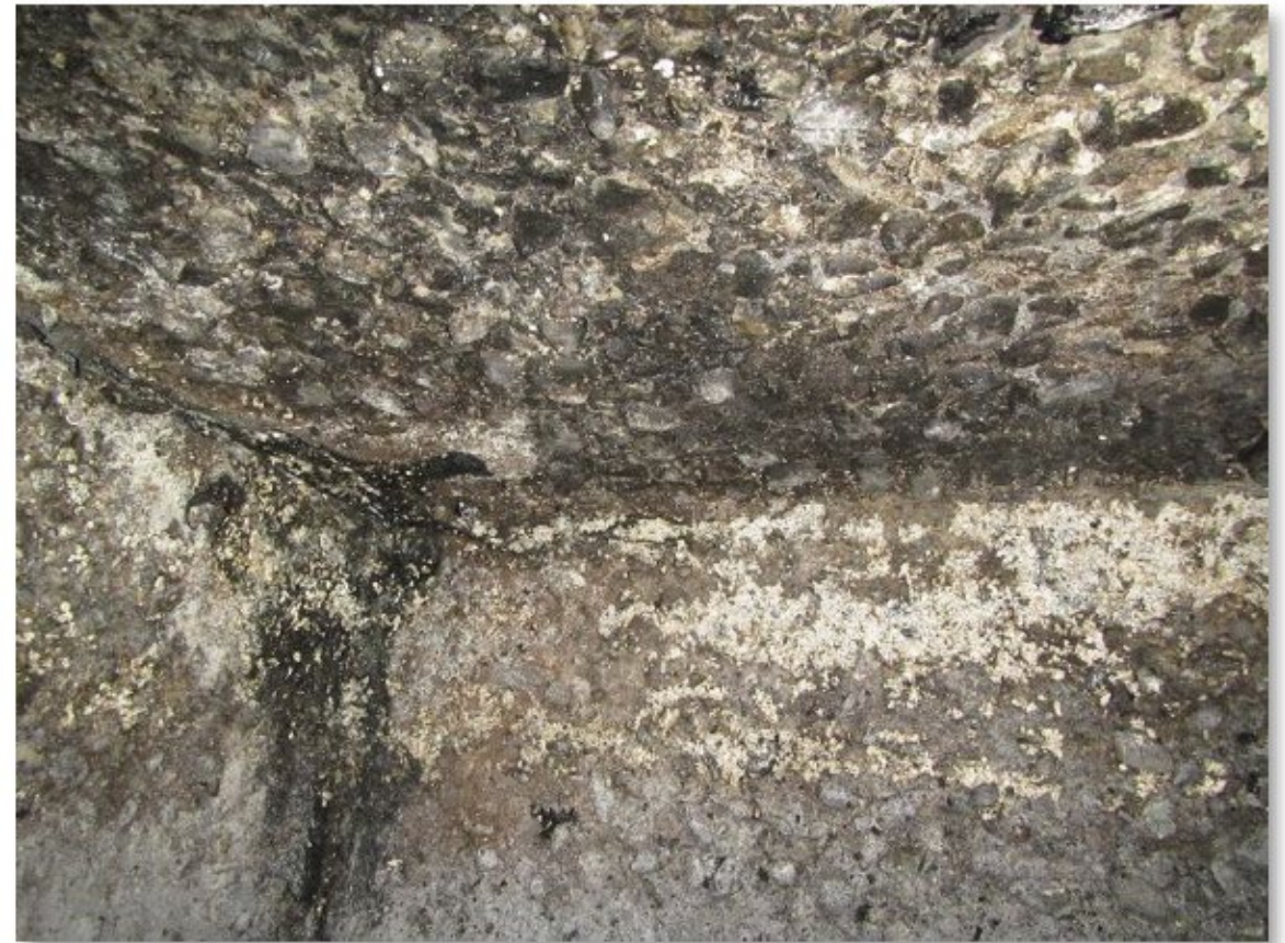
Photo 3-20. Wall and ceiling of JB4 with large aggregate exposed.
