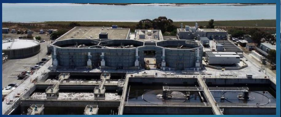
Critical part of secondary (biological) treatment process All 3 FFRs in need of rehabilitation Structural, Mechanical, & Electrical aspects
