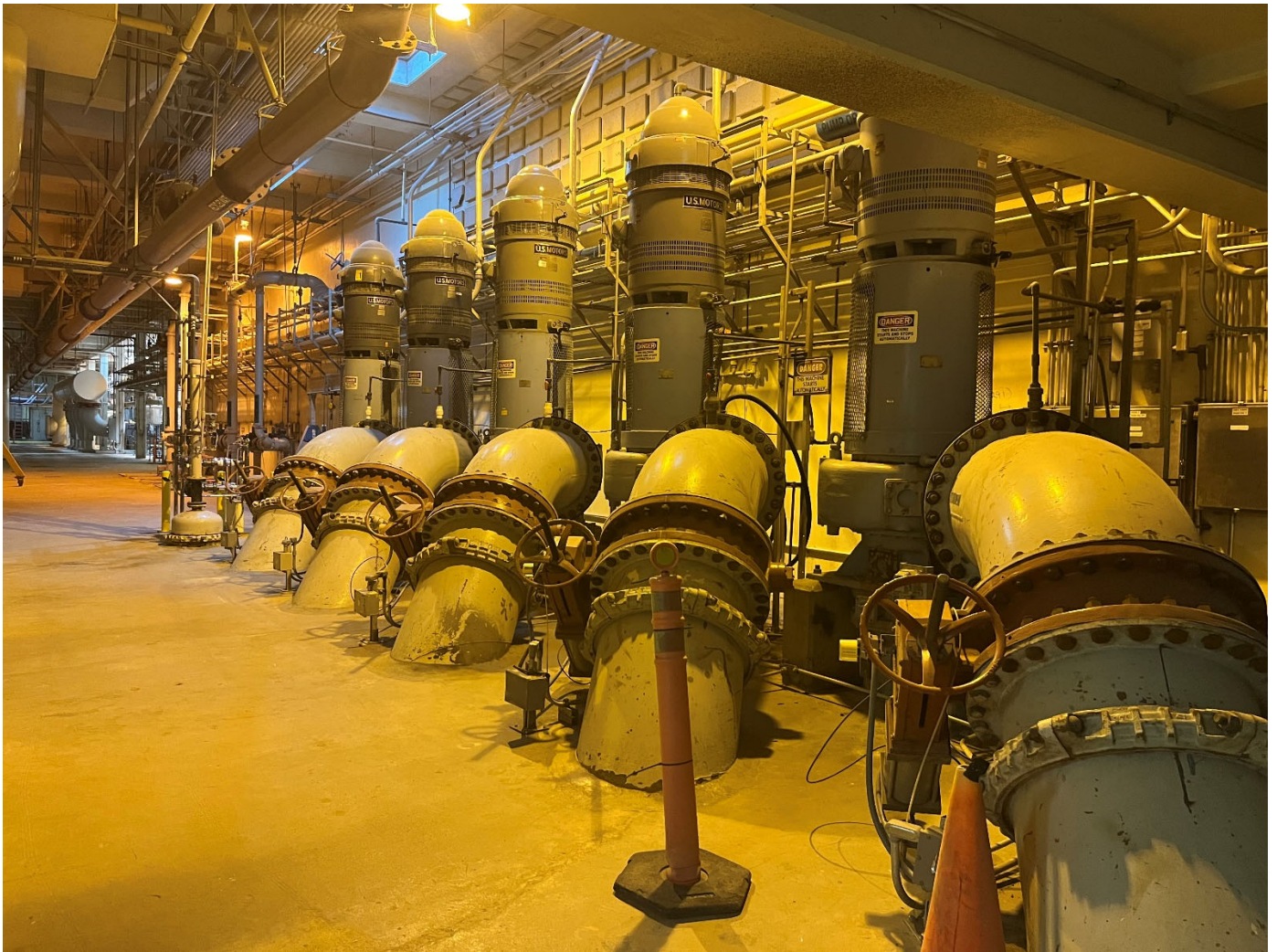
Figure 1. SVCW Final Effluent Pump Station
