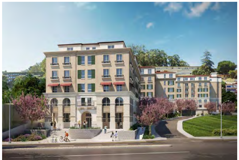
800-803 Belmont Avenue – 125-unit all-affordable residential apartment development (currently under construction)
