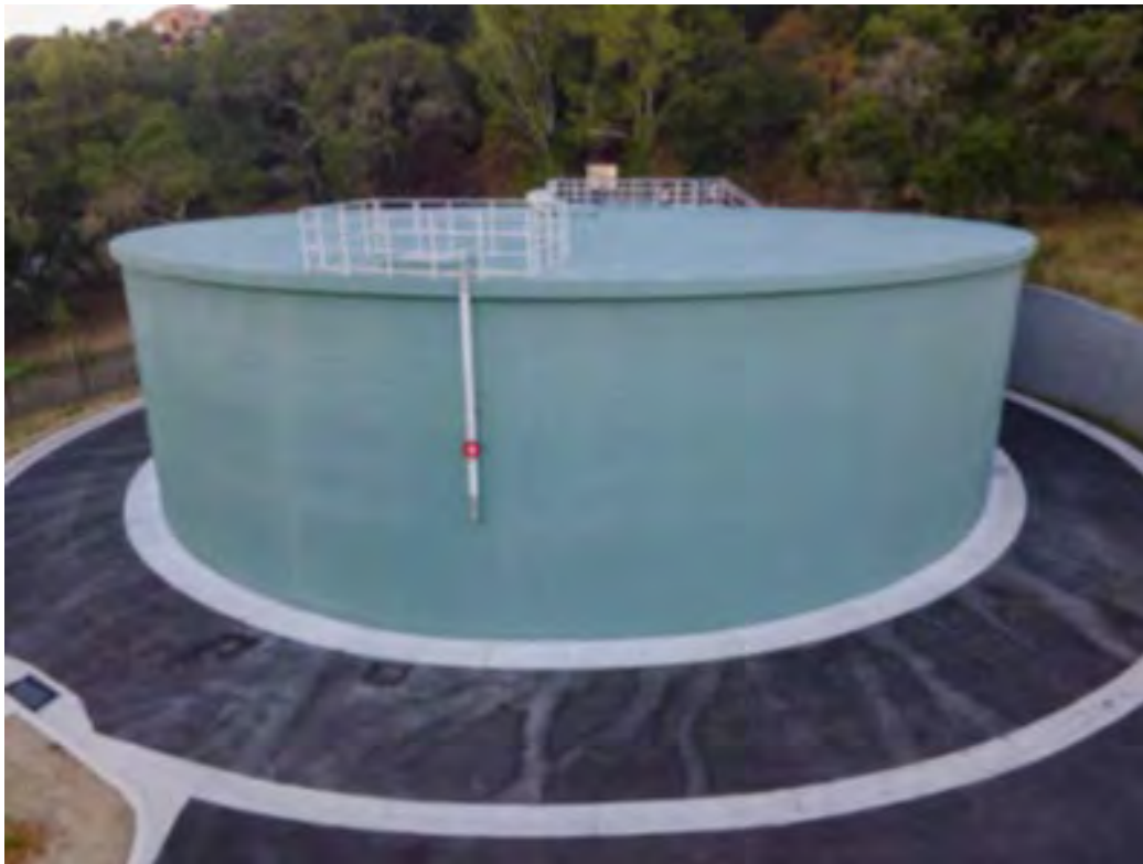
California Water Tank
