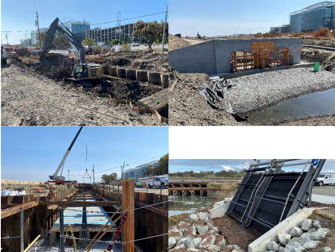
Construction photos from the Bayfront Canal & Atherton Channel Flood Protection Project
