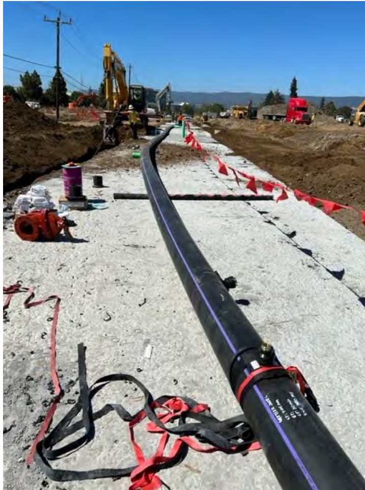
1548 Maple Street Pipeline Extension
