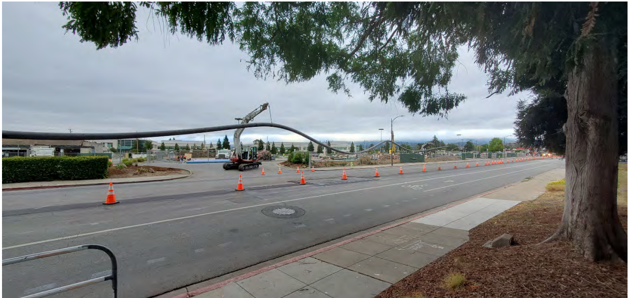
Broadway Plaza Pipeline Extension
