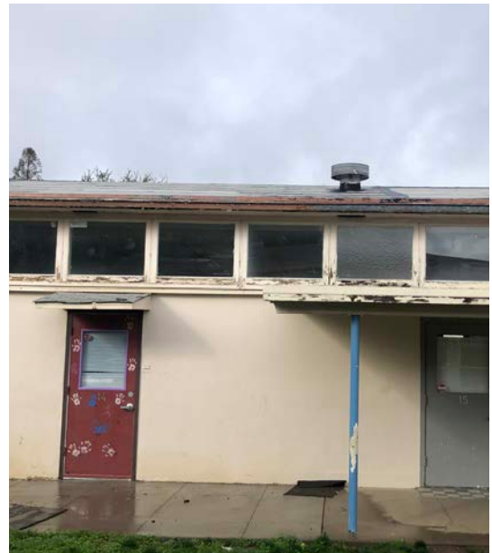
75-year old aging Barrett Community Center
